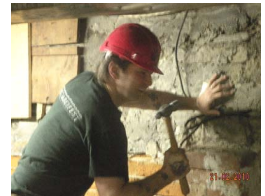
Volunteer Glen Mackey from Newfoundland completes necessary repairs in our basement.
